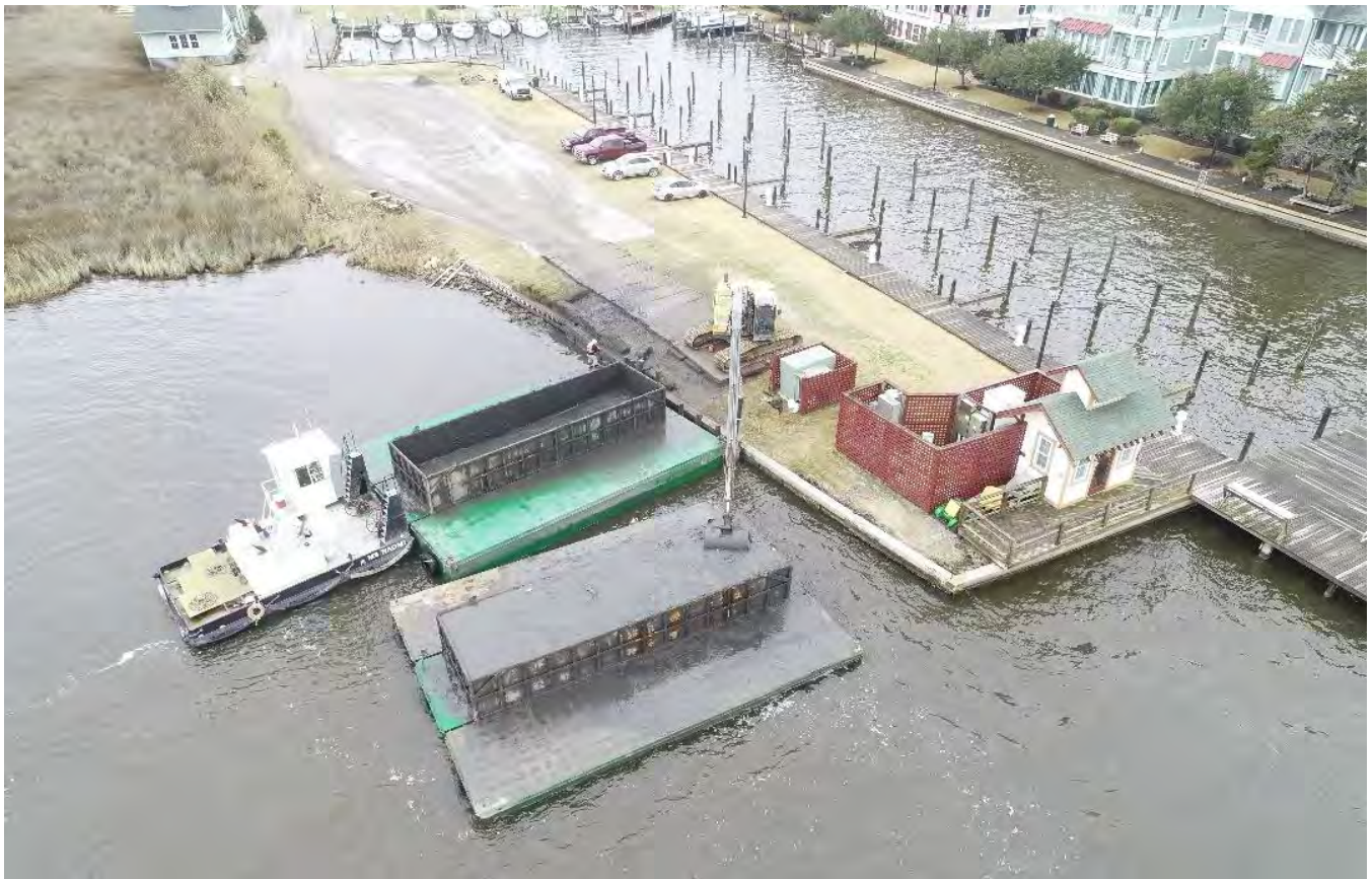
(Above) Photo 7: 2021 Mechanical Dredge Transfer Station, Shallowbag Bay, NC. Source Credit: Dare County Grants and Waterways
